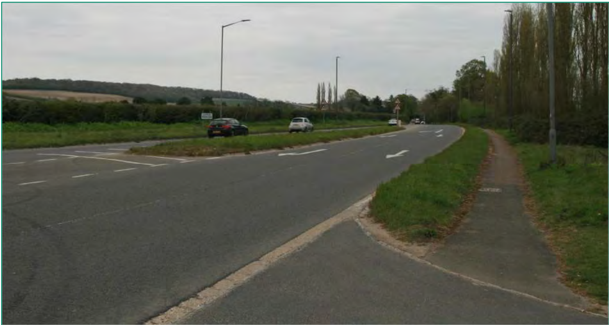
Figure 2-8: Photo of A4155 Marlow Road Eastbound (21 April 2021)
