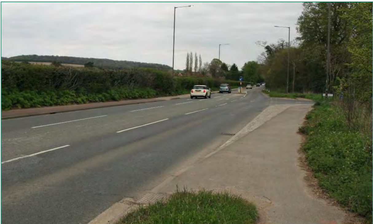
Figure 2-9: Photo of A4155 Marlow Road Junction with Westthorpe Farm Lane (21 April 2021)
