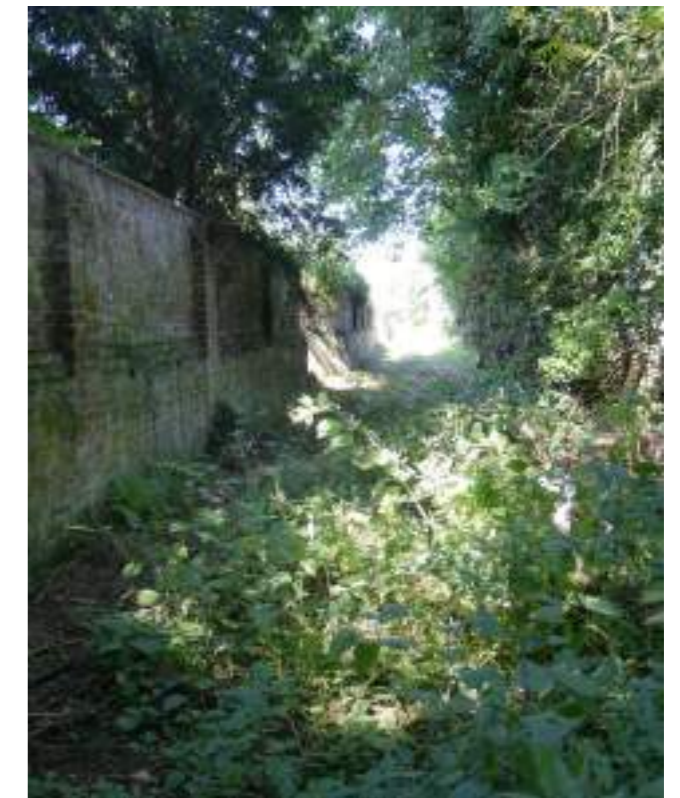
Figure 8.15 Garden wall around Westhorpe Park Homes
