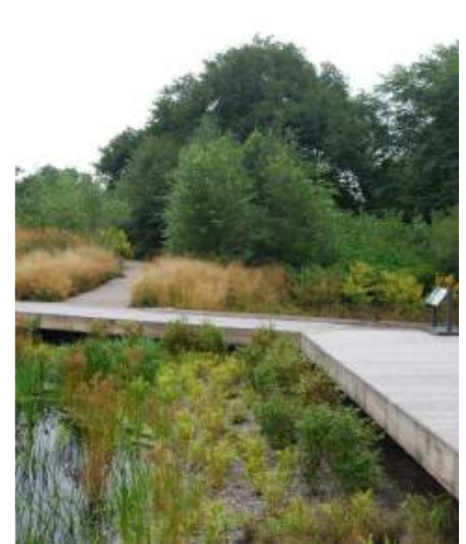
Figure 8.78 Sustainable Urban Drainage attenuation planted for ecological value
