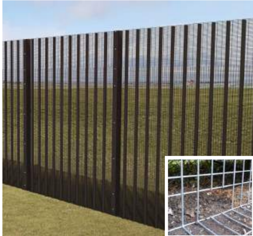
Figure 8.123 2.4-3m height 358 weldmesh fence with wildlife access panels
