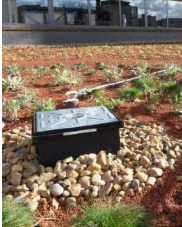
Figure 8.132 Blue roof storage
