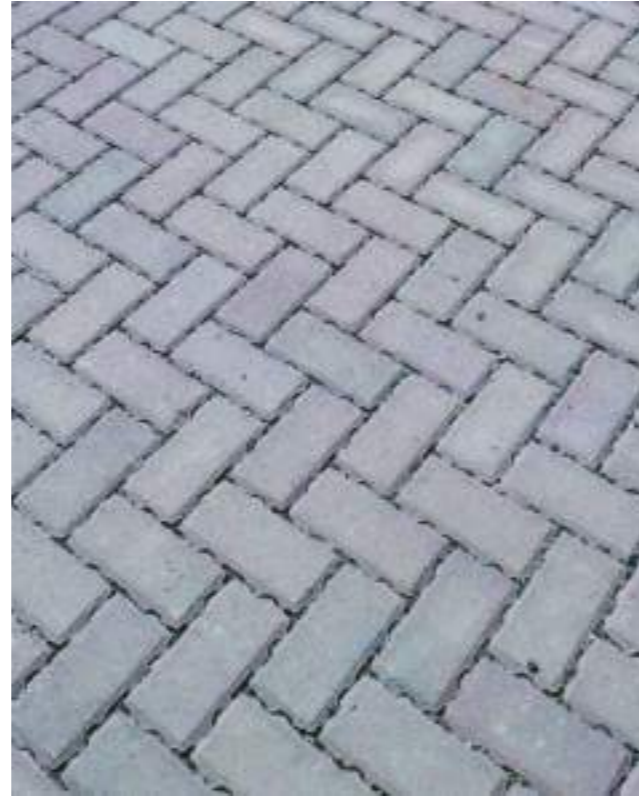
Figure 8.133 Permeable block paving
