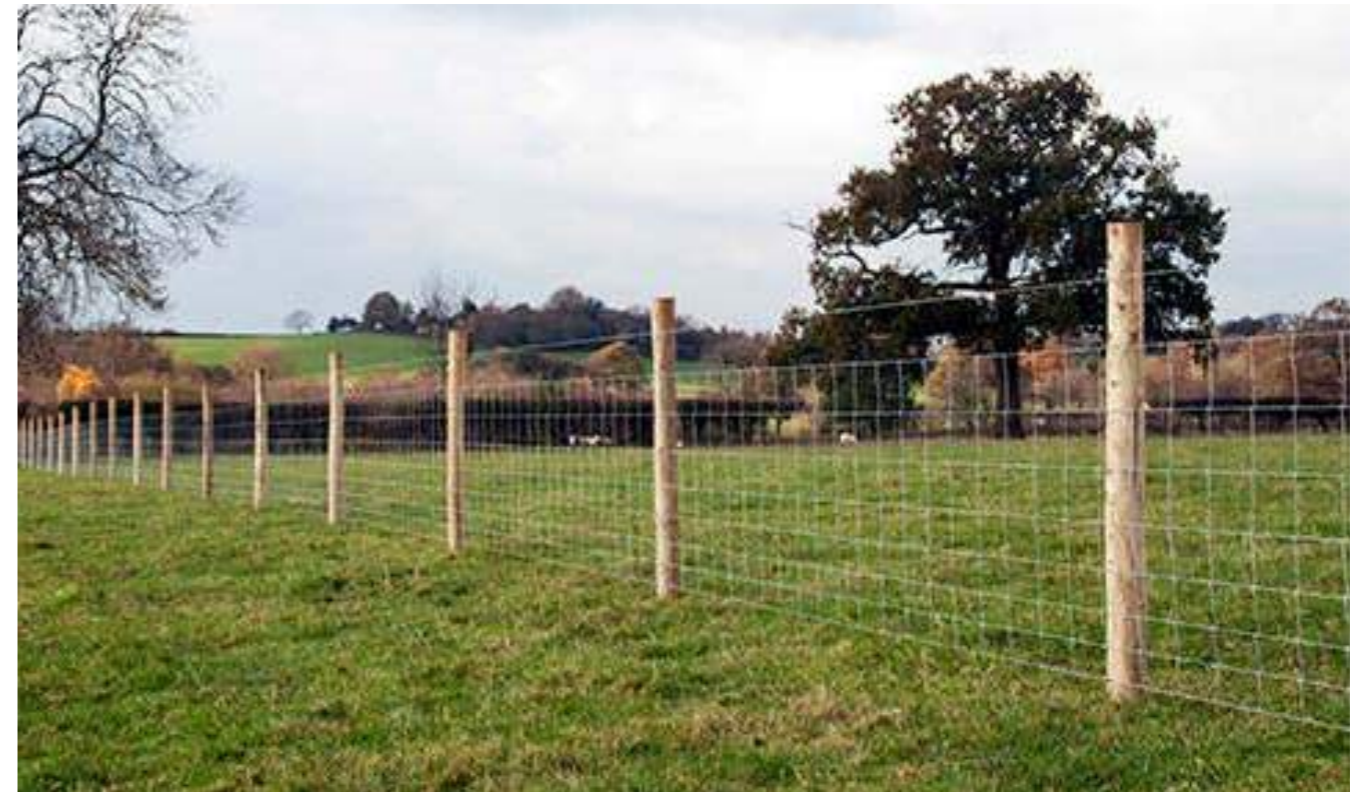
Figure 8.128 1.2m sheep fencing to Plot 5
