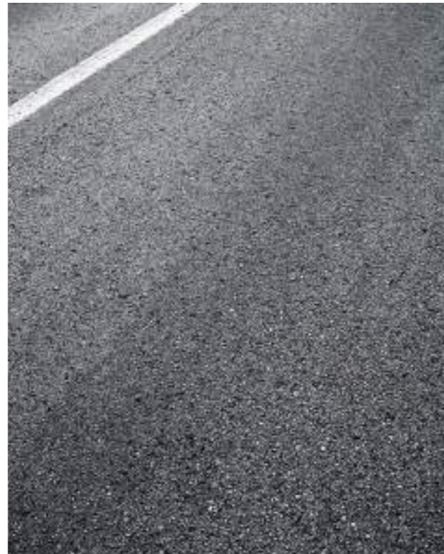
Figure 8.112 Asphalt to carriageways
