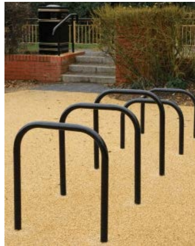
Figure 8.120 Kerbside cycle stands
