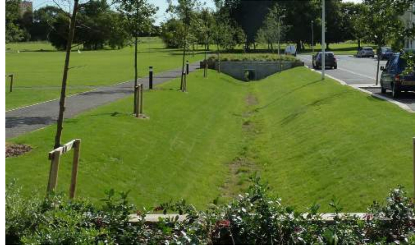
Figure 8.134 Biofiltration strips in streets
