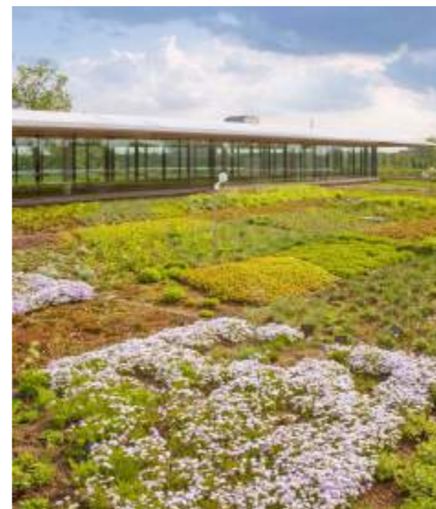
Figure 9.15 © Green roof Rice Plant Conservation Science Centre © Daniel F. Ada. L
