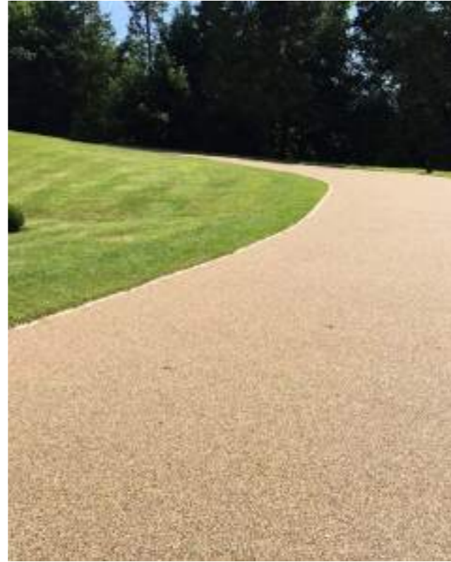
Figure 8.109 Resin bound gravel footways
