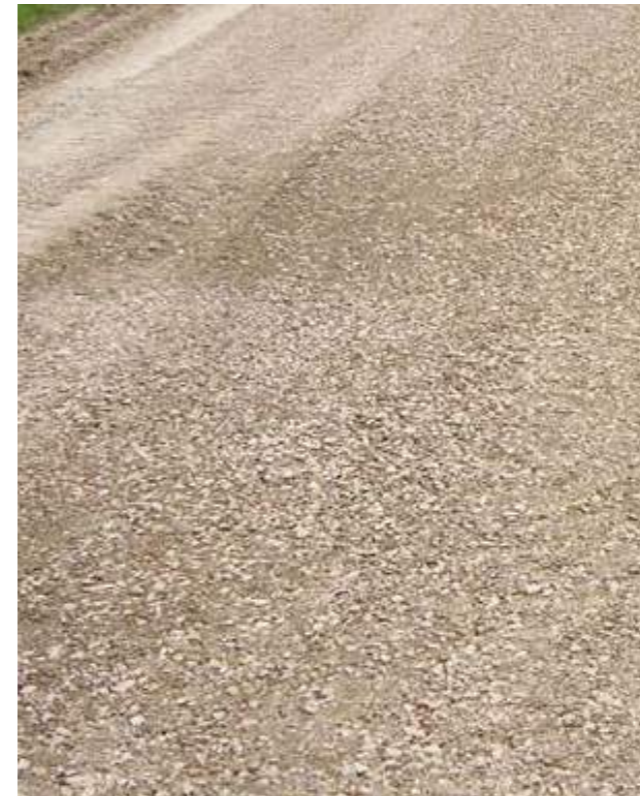
Figure 8.113 Compacted gravel to tracks and backlot
