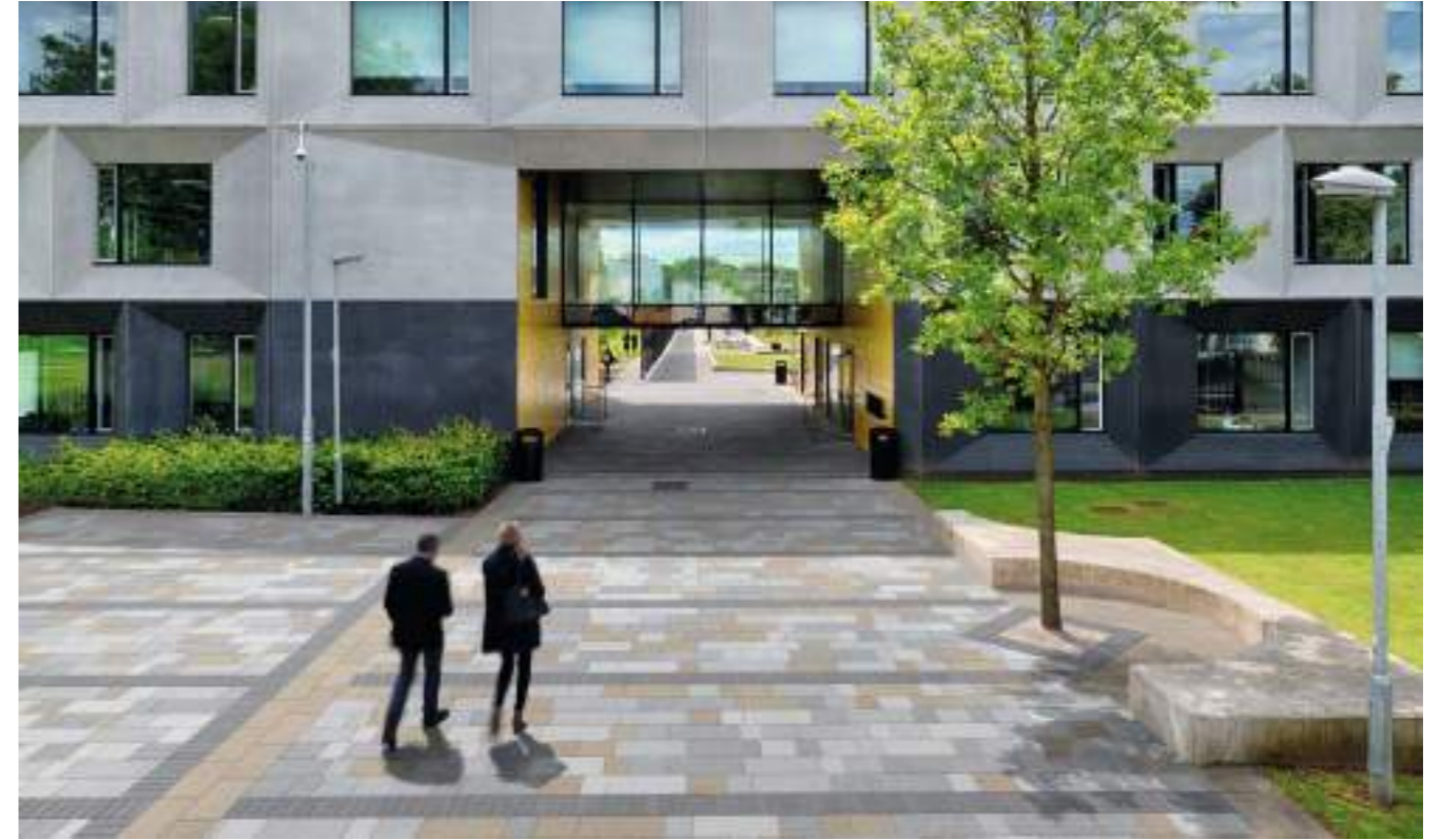
Figure 8.110 Concrete setts to focal spaces / pedestrian spine
