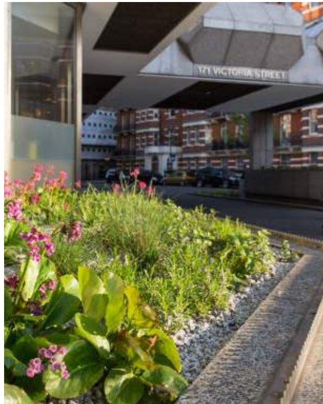
Figure 8.135 Rainwater planters along buildings
