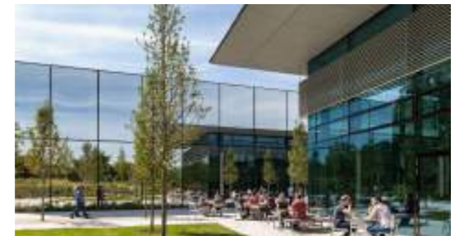
Figure 6.51 Dyson Campus © WilkinsonEyre 2022
