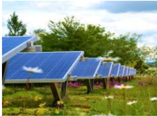
Figure 6.122 Green flat roof with PV panels © Contec
