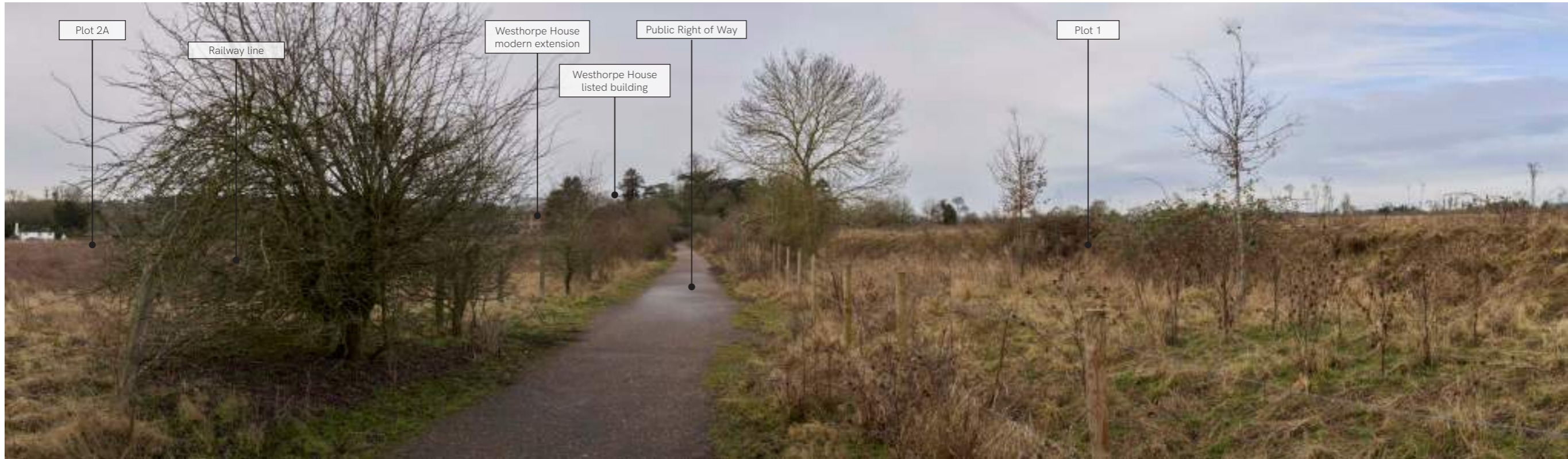
Figure 5.41 View 12 from the Public Right of Way looking west. The unfinished extension to Westhorpe House is partially visible whilst the listed building is almost completely concealed within dense tree canopy
