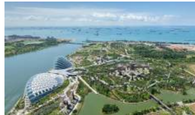
Figure 1.4 Cooled Conservatories, Gardens by the Bay
