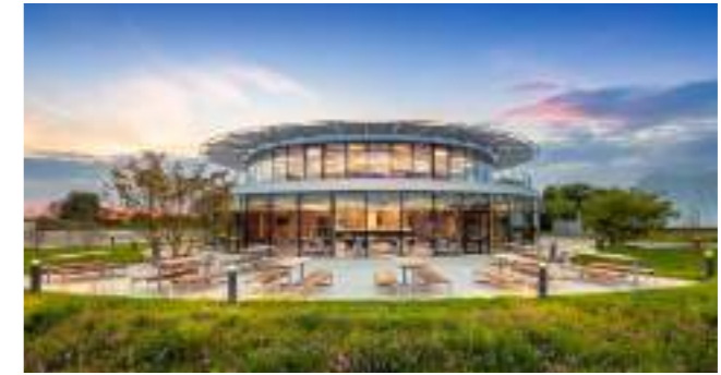
Figure 6.50 Dyson Campus © WilkinsonEyre 2022
