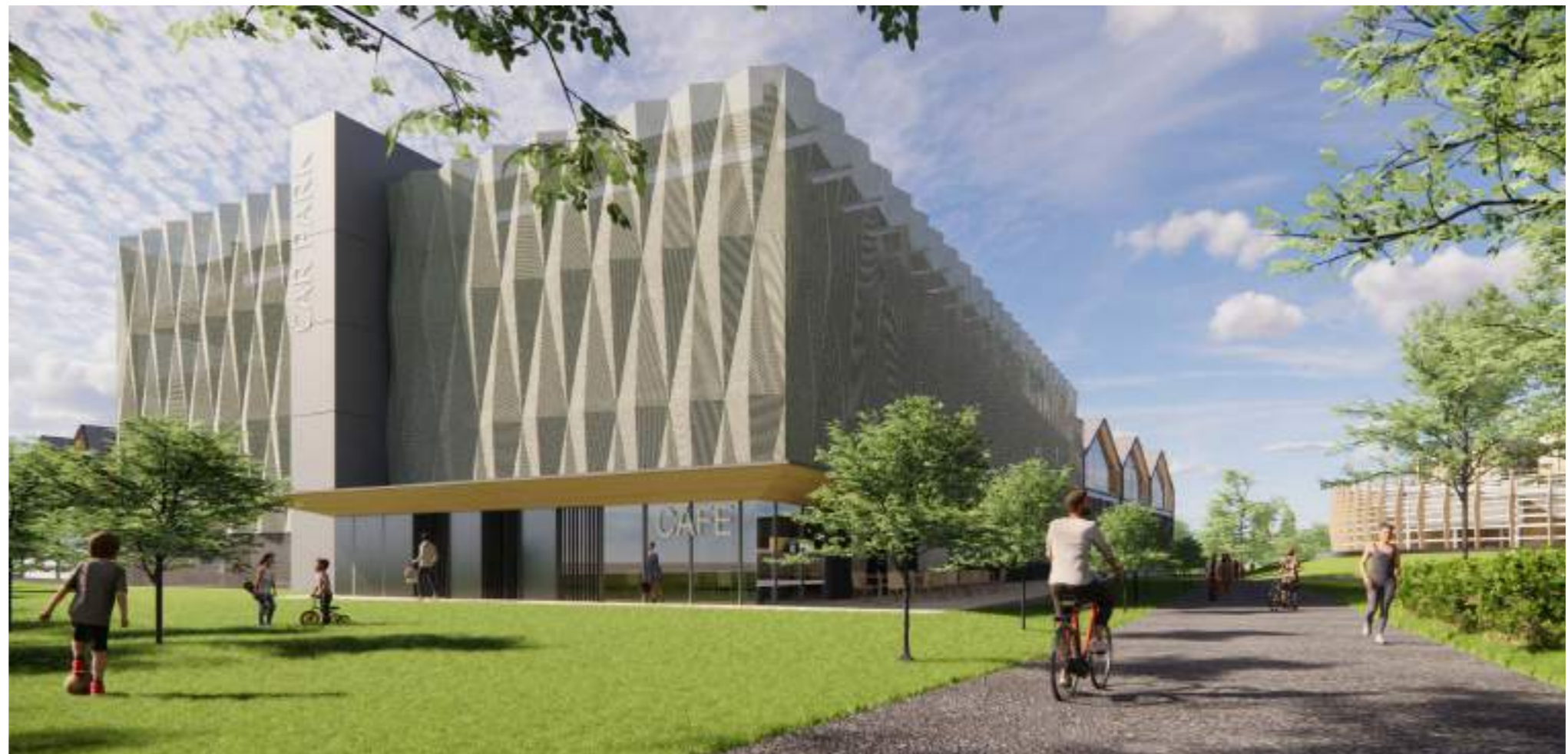
Figure 7.106 Southern Multi-Storey Carpark View from the East along Public Right of Way
