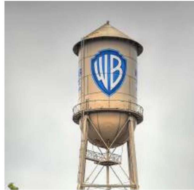
Figure 7.126 Warner Brothers Water Tower
