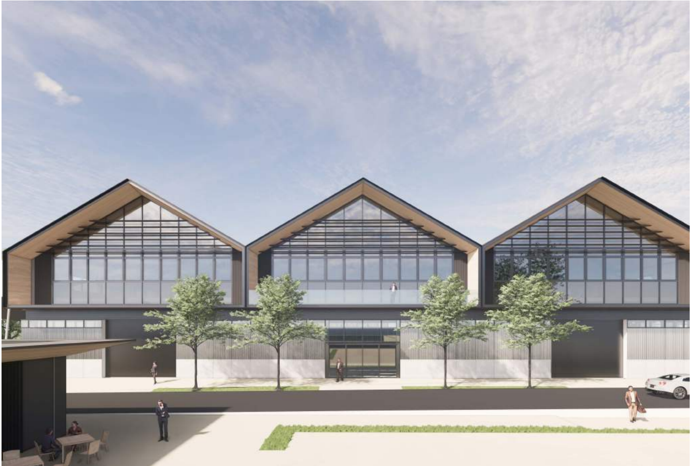
Figure 7.62 Workshop & Office Primary Facade View
